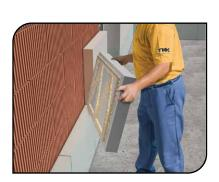
**Tekapur Insulation Adhesive** hand held is a low-expanding one-component polyurethane adhesive used for mounting insulating materials. It is hardened by air humidity.
